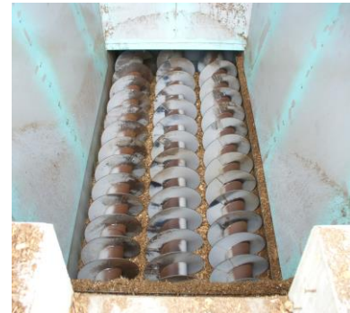
Mounting in discharge screw (wood-fired power plant)
