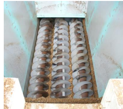
Mounting in discharge screw (wood-fired power plant)
